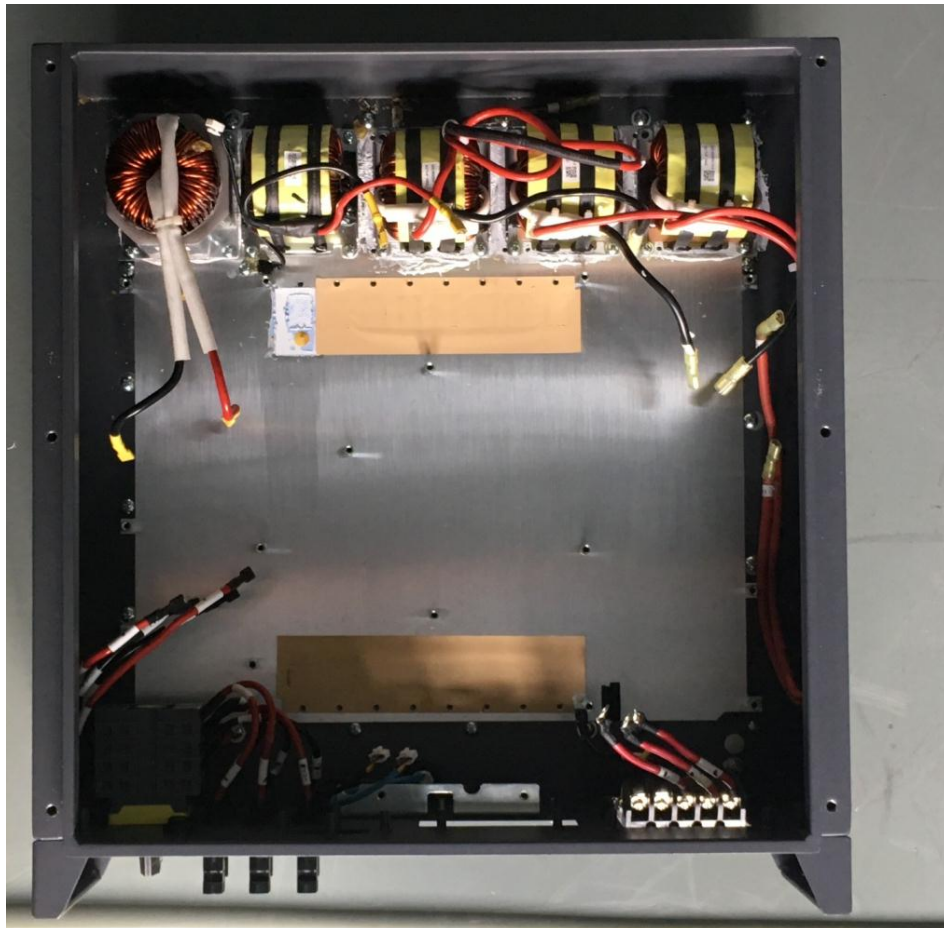
Checked after test finish
